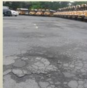
Cambria, Technology Pave/overlay asphalt parking lots
