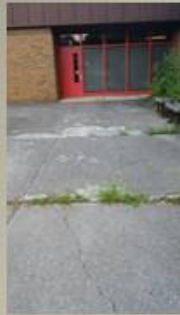
GLE, FBE, HAE Replace concrete sidewalks
