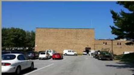
CHS and SMS Brick masonry improvements for serviceability - CT
