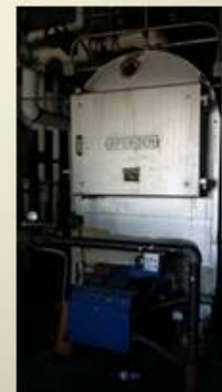
CPS Install new boiler - CT
