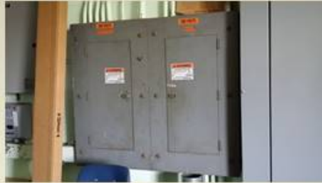
BES, GLE, MBE, CES and SMS Replace select electric panels
