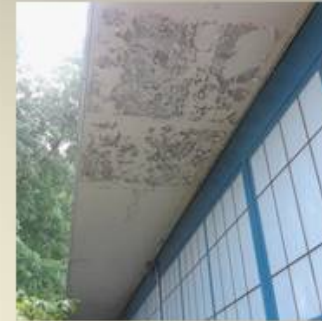
CES, MBE, GLE Replace ACM soffit – CT/CMPL
