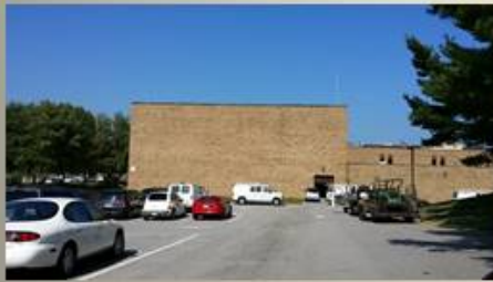
CHS and SMS Brick masonry improvements for serviceability - CT
