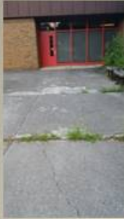
GLE, FBE, HAE Replace concrete sidewalks
