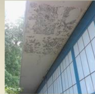
CES, MBE, GLE Replace ACM soffit – CT/CMPL
